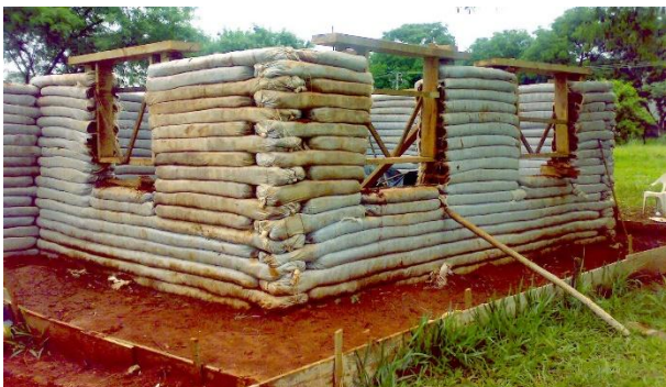
Picture 9 - Construction of self-supporting orthogonal earthbag building
