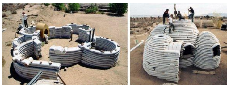
Picture 7 - constructions of self-supporting superadobe domes
