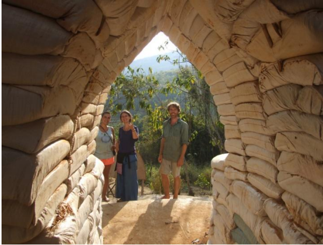
Picture 8 - Superadobe gothic arch as a small entrance corridor
