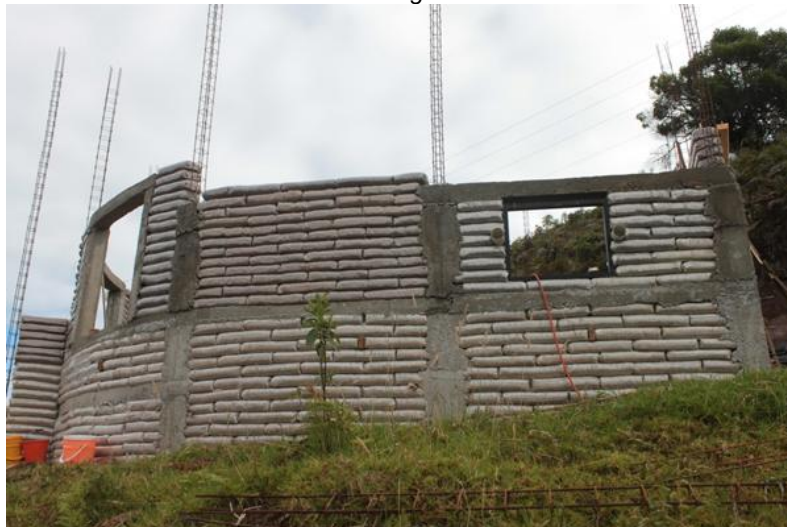
Picture 15 – Detail of a confined earthbag construction with reinforced concrete
