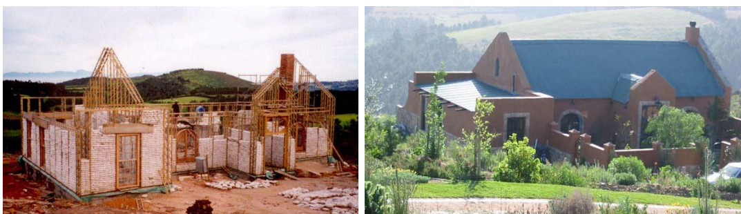
Picture 11 – Before and after of a sandbags constructions with Ecobeam construction
