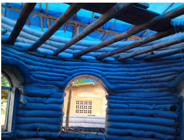
Picture 3 - Construction of 2 nd floor of Majestic Dome, Panamá.
