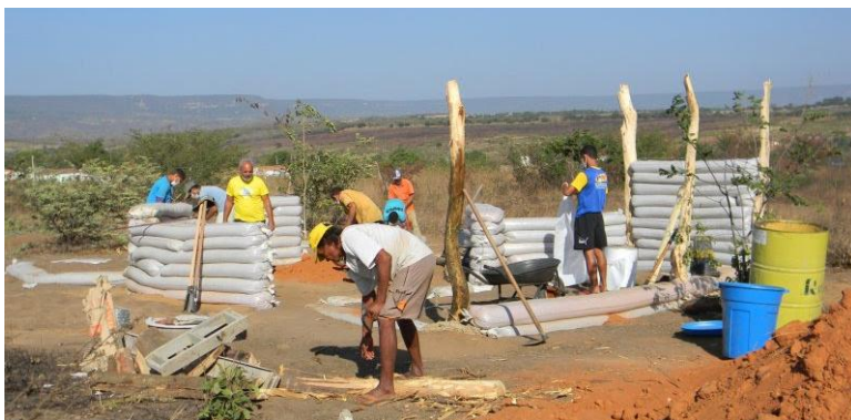
Picture 10 – Superadobe construction with timber structure in Ceará, Brazil.
